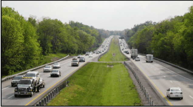
Figure 4. I-71 Northbound Approaching I-265
